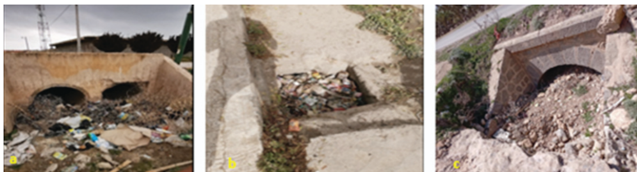
Figure 8. Malfunctioning of the urban drainage system observed in the field: (a) Heavily loaded discharge canal, impairing proper flow. (b) Sewer blocked by solid waste, observed in a residential neighborhood. (c) Drainage structure clogged with poorly sorted coarse sediment deposits (silt, gravel), hindering flow and promoting overflow.
