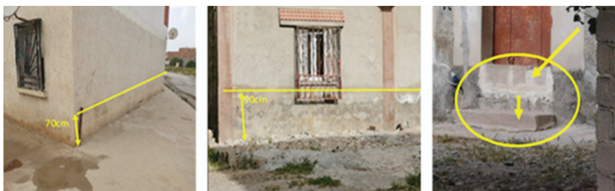
Figure 11. Effects of the June 2023 flood on buildings and residents' individual adaptations: (a, b) Flood marks visible on the walls of a dwelling (June 2023). (c) Raised doorway threshold installed to limit water intrusion.
