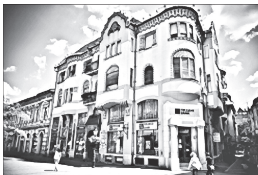
Picture 2. Subotica Savings Bank Palace
