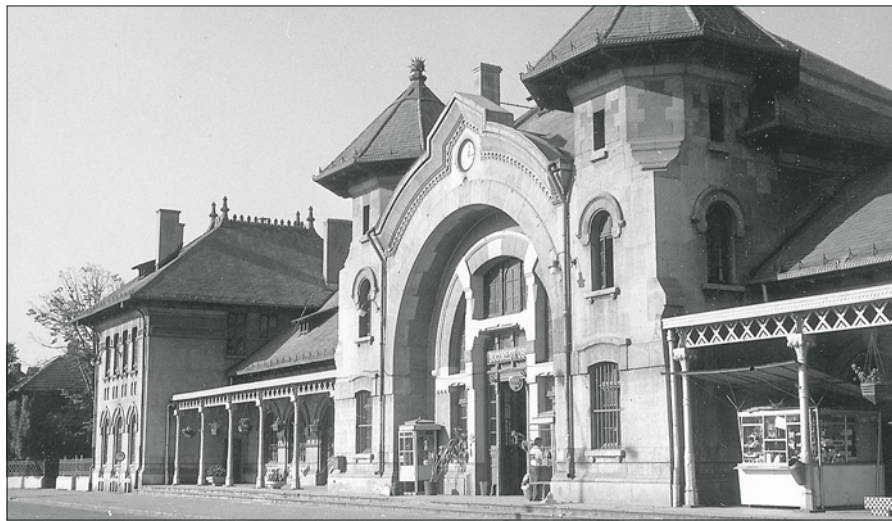
■ Plate 5. The new station of Bucharest Obor built in the 1930s
