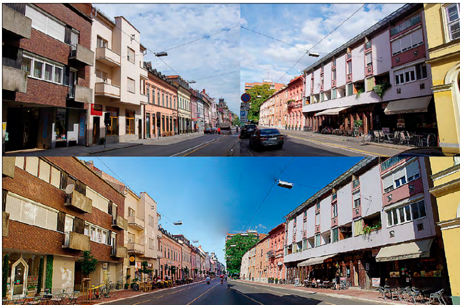
Figure 9. The panorama of Oskola Street (odd-numbered and even-numbered houses) from the south. Photos by Karancsi and Hornyák
