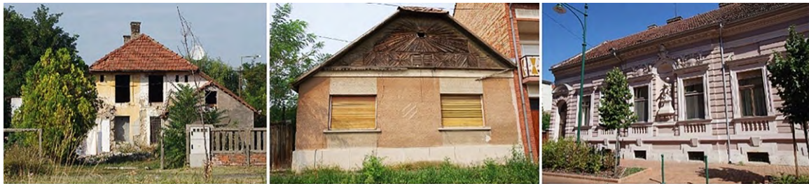
Figure 2. The determination of core values on the basis of the physical condition of buildings (from left to right): very bad (1 point); average, with some clearly visible aesthetic problems (2 points); a renovated building in perfect condition, (3 points)
