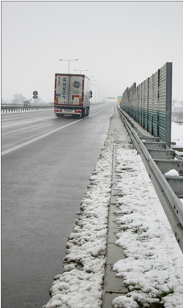
Figure 7. Noise barrier wall at the Dobanovci interchange keeps snow in front of panels - NS-BG direction Source: Ivana Sentić
