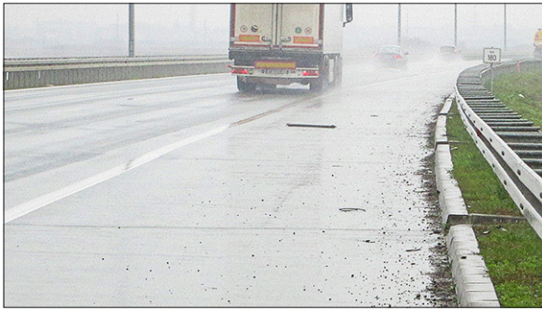
a. Immediately after the Dobanovci interchange in the vicinity of Batajnica – influence of rain and strong wind, good conditions for deposit of soil materials on the highway, BG-NS direction
