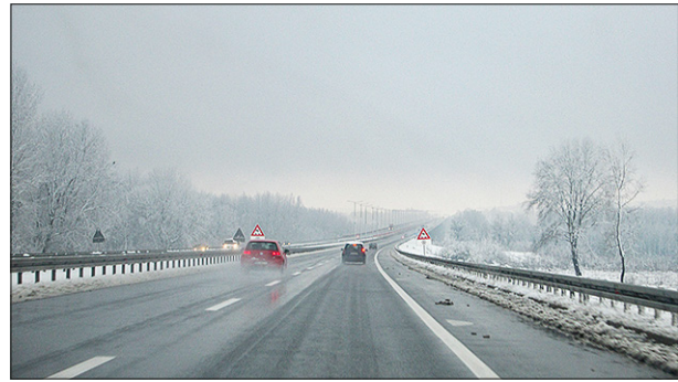
b. Beška Bridge - snow and frozen snow deposits on the highway, NS-BG direction. Deposits could be from the adhesion on vehicles or the influence of wind
