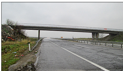
a. Dumpsite near Batajnica - BG-NS direction
