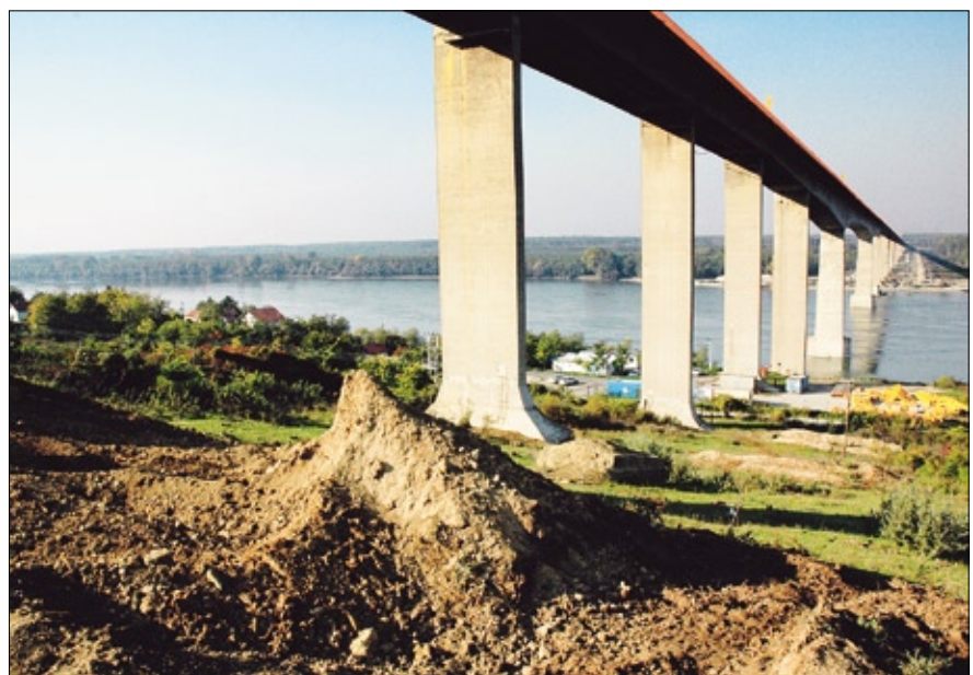
Figure 5 The southern edge of the E75 highway bridge near Beška (18.10.2007)
