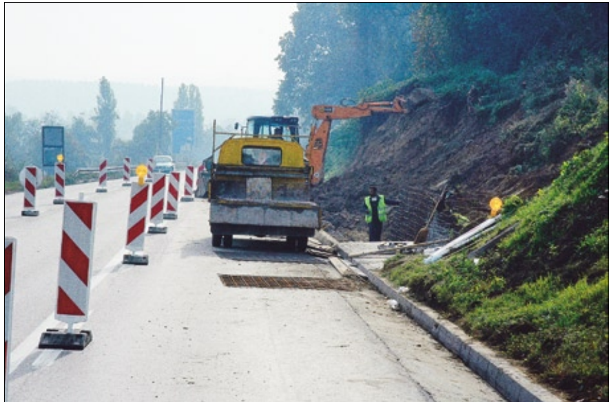
Figure 1 Repair work on a section of the Beograd- Novi Sad regional motorway near Sremski Karlovci (18.10.2007)
