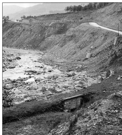
■ Plate 17 The Basca valley near Gura Teghii showing how the CFF trackbed was completely washed away in places (1976)
